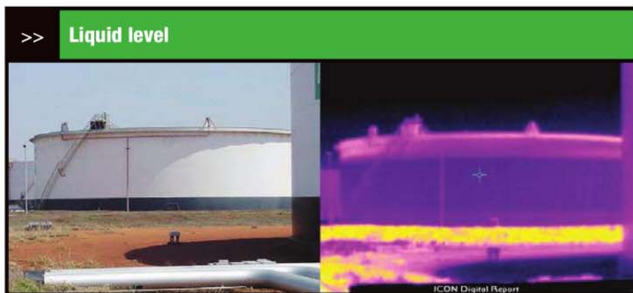
Figure 1. Thermal image clearly indicates the level of fluid within the tank. Source: Fluke
