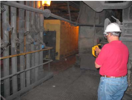
Below: Inspecting boiler drain lines
